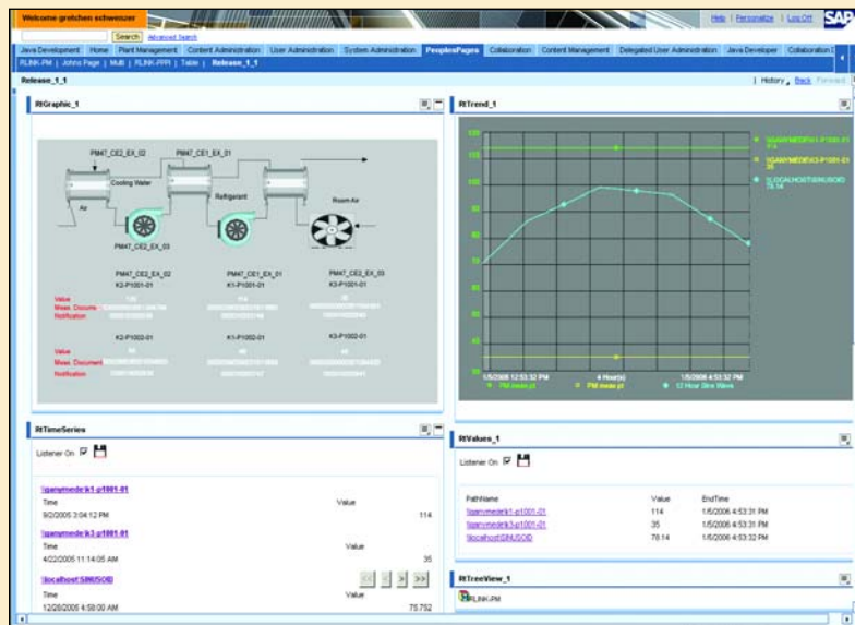
FIGURE 1 ▲ The OSisoft PI System gathers operational data from across the enterprise and, through Facility Monitor, displays this information in common application front ends, like SAP NetWeaver's portal
